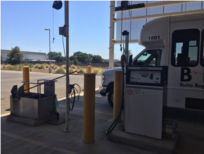
Vehicle fuel island and probing station.
